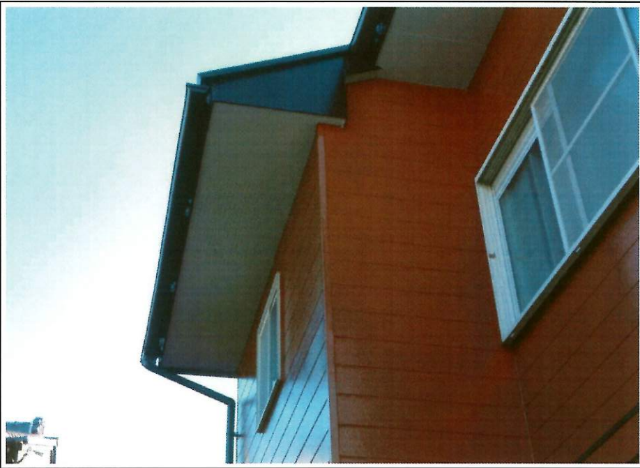
③8外壁 AFTER
