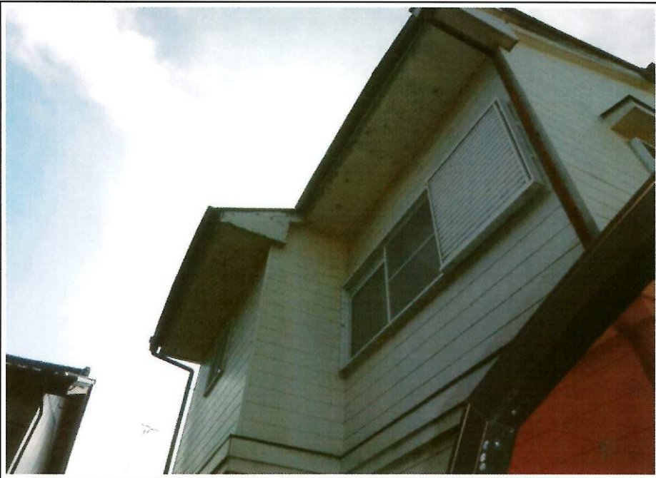
③7外壁 BEFORE
